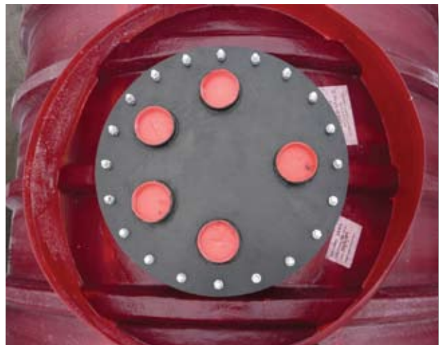
Manway Cover, Fittings & Vacuum Monitor
