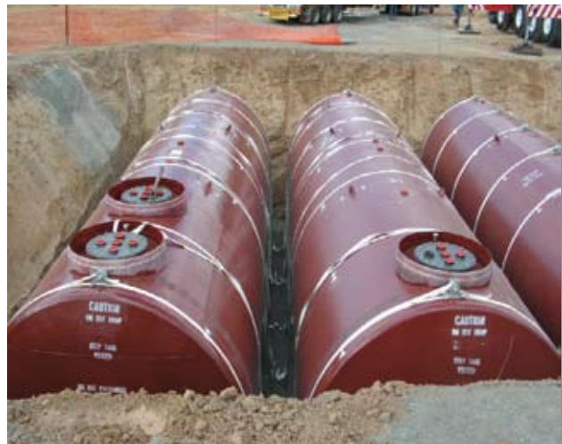
FTS Tank Strapping & Anchor System
