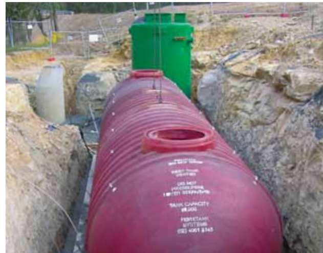
Mullaly Lift Station with 110,000 litre Emergency Storage Tank 2.750 diameter x 7.000 deep & 6.000 deep
